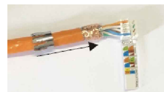
6.Cut the extra wires until the horizontal line.Move the screw on the top of copper foil paper.
