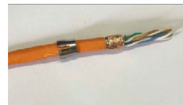
4.Make copper foil paper winding on the earth grounding wire.
