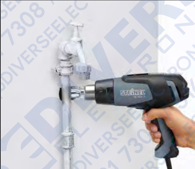
Thawing frozen pipes.
