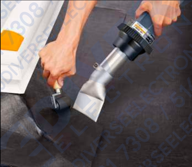
Overlap welding on a light dome.
